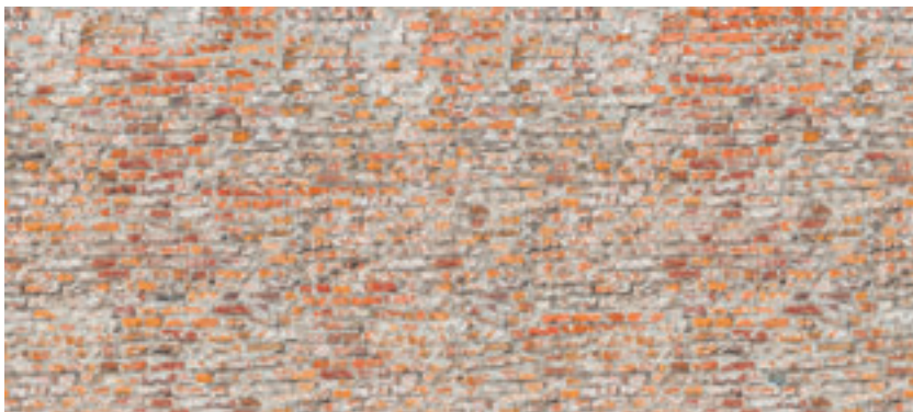
G1-05-05 • Worn Brick • Worn Brick
